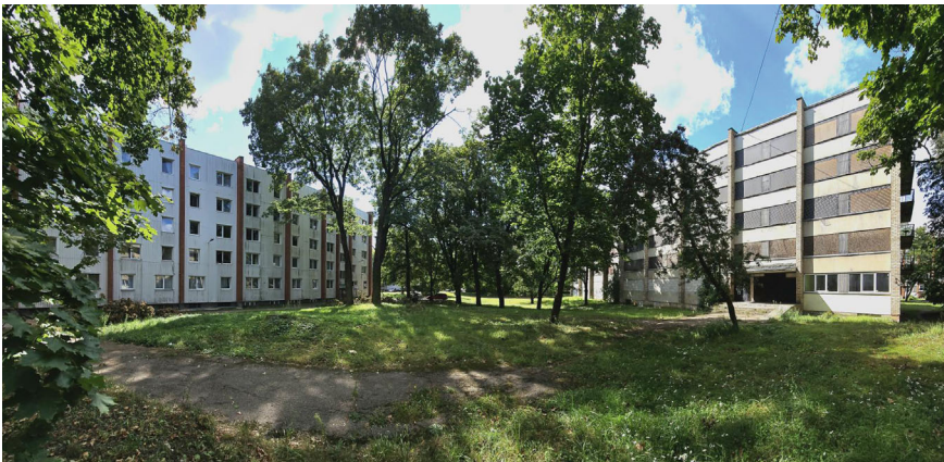
Fig. 1 Formerly renovated Ziepju 13 (left side) and the abandoned Ziepju 11 (on the right)
